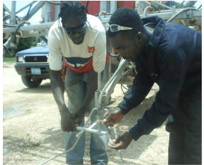
*Checking & adjusting spray nozzles*
