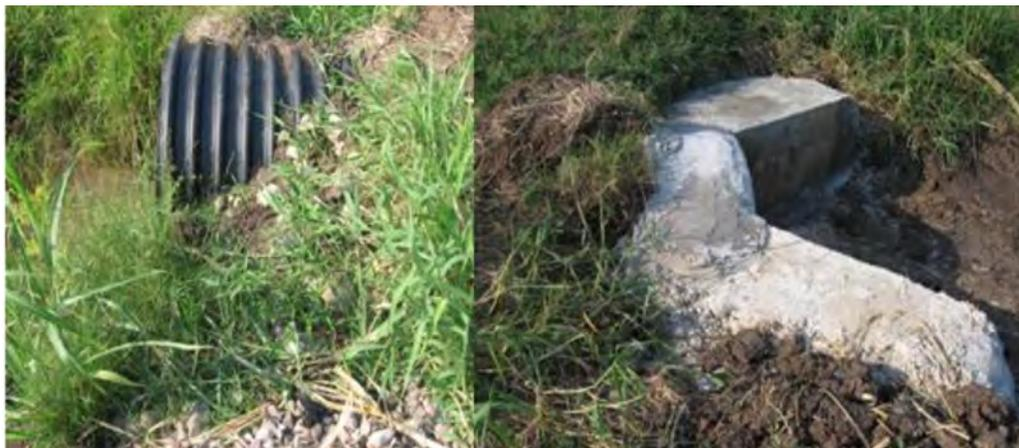
Fig. 2: Ribbed Polyethylene Pipe used for Culvert Crossings
